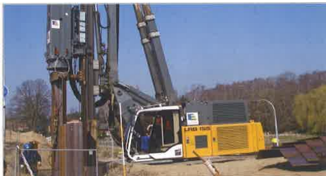
Integrated Driven Piling Rig with Hydraulic Hammer 液压锤驱动打桩机
