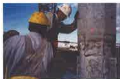
Sure Lock Mechanical Pile Splice for Precast Pile Segment 预制桩段的锁紧机械桩接头
